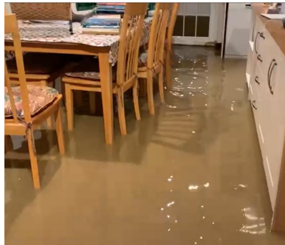
Figure 10: Video still of Internal flooding to No. 8 Blackmile Lane on Sunday 22 Sept 2024. NOTE water entering via door in background. (c) R. Blacklee
