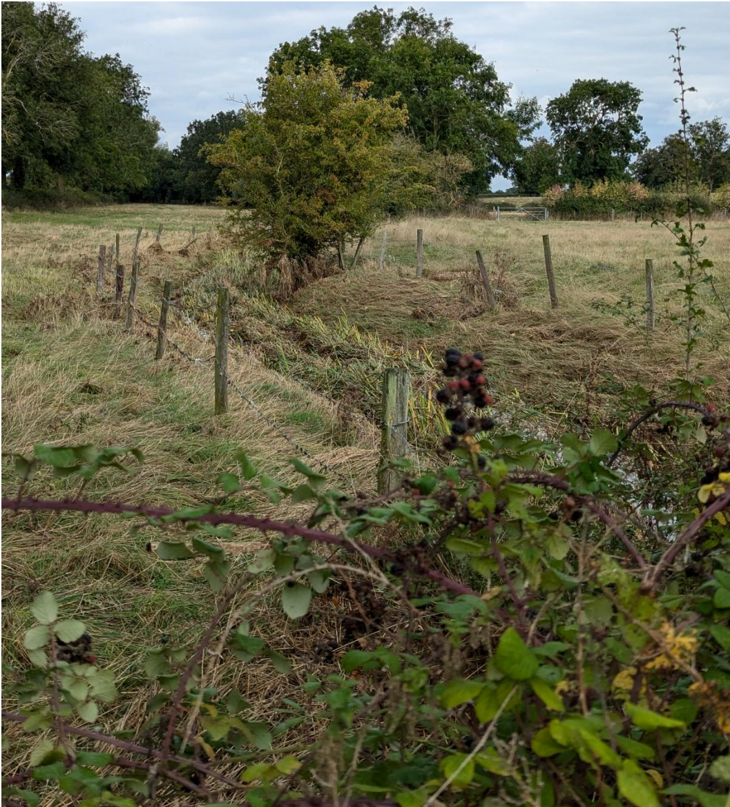
Figure 20: Obstruction J on Gbbards Arm showing overgrown channel banks and bed. © C. Dow
